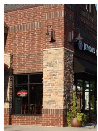
Not acceptable because the stone pier does not continue to grade and the surface below the glazing repeats the brick.
