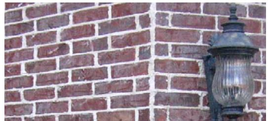
The mortar color will be darker emphasizing the brick. The mortar above is not permitted.
